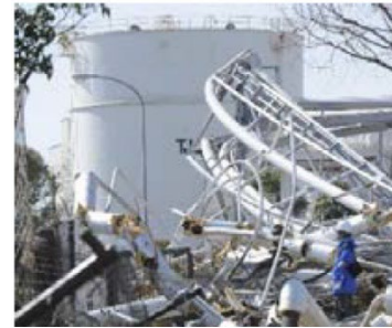
Sendai Minato Gas Plant
