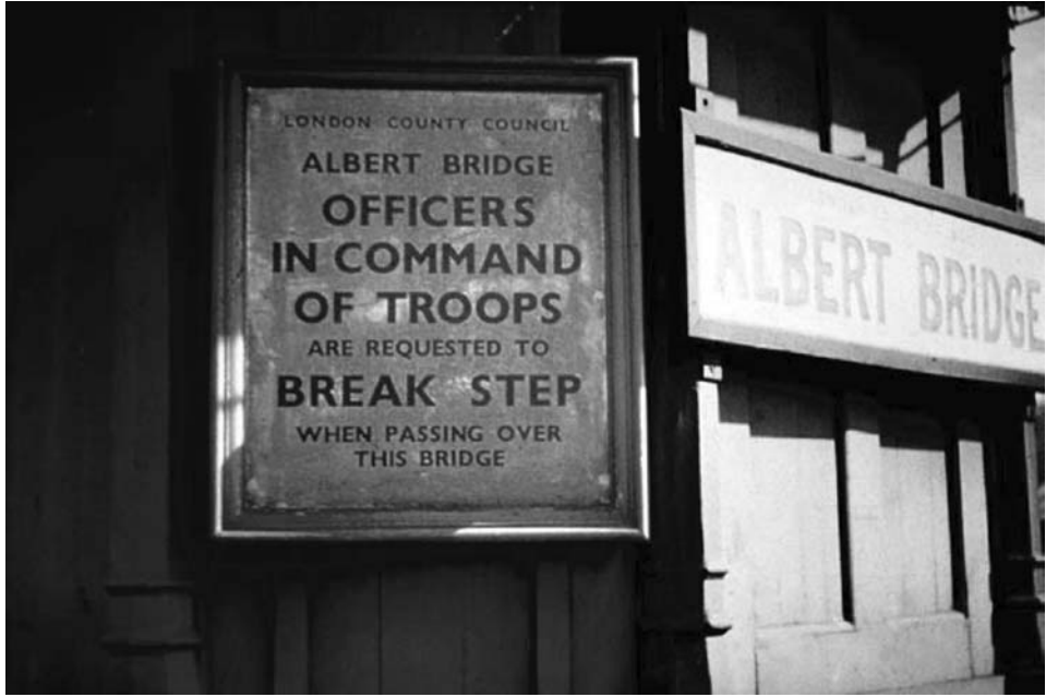
Fig. 15.4. A sign on the Albert Bridge in London, instructing troops to break step to prevent destructive resonance effects. (Courtesy of the National Information Service for Earthquake Engineering, University of California, Berkeley.)
